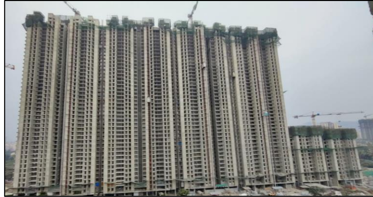
Tower No 1 - 5 – Current picture
