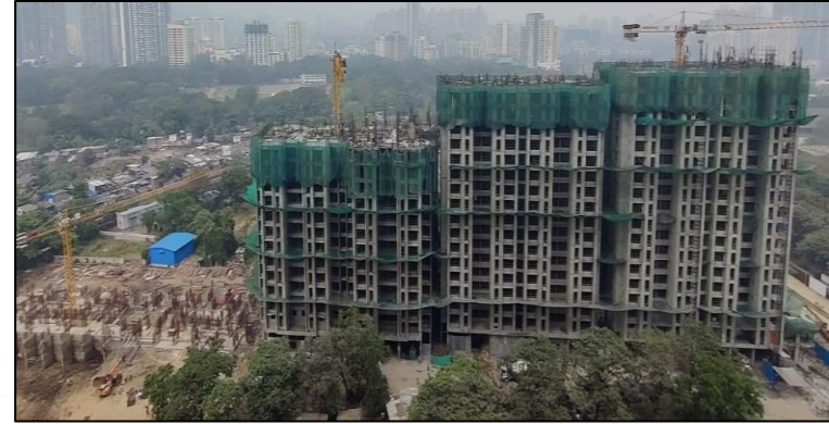
Tower No 6 -10 – Current picture
